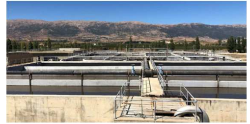
Jeb Jenin Wastewater Treatment Plant
