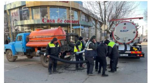
Coaching in Sewer Network Cleaning, 2024
